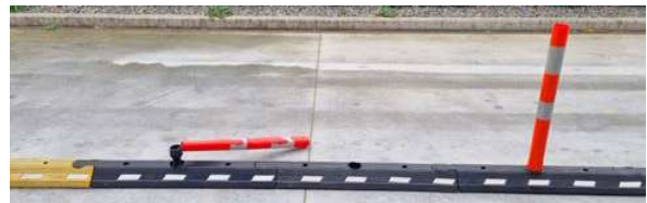
Left: Old plastic post broken after 30 x hits. Right: New post still looks brand new after 30 x hits.
