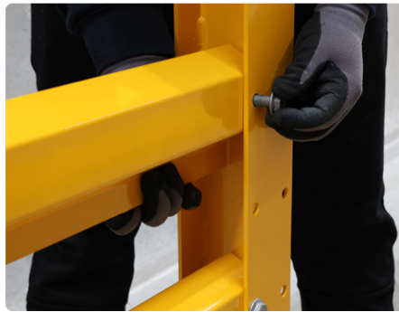
▲ Insert rails into posts and secure with bolts
