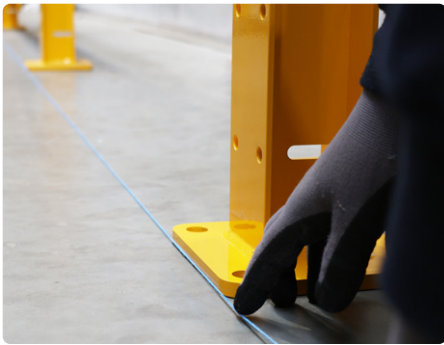
▲ Run a string line from the first to last post
