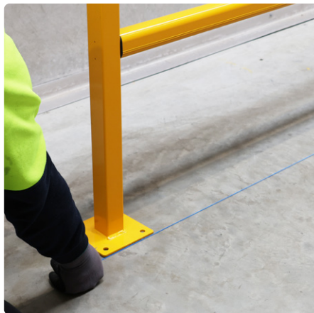
▲ Use a string line to straighten the run
