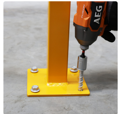
▲ Fix posts with concrete screws
